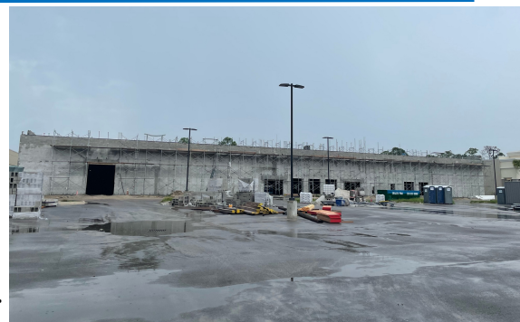
Building continues on the new Publix – it is starting to look like a Publix!
